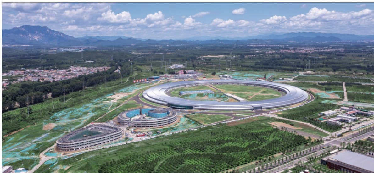
View from above The ground-breaking ceremony for the High Energy Photon Source (HEPS) took place in 2019, with the linac and booster installation now nearing completion. The storage ring will be completed in 2023, with the first synchrotron X-rays expected in 2024.
